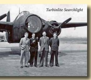
bombers available during the conflict, and employed its Bostons largely in night fighting and ground attack roles. One of the most unique variants was the Turbinlite modification, which essentially turned the aircraft into an enormous flying flashlight for use in illuminating German bombers at night.
